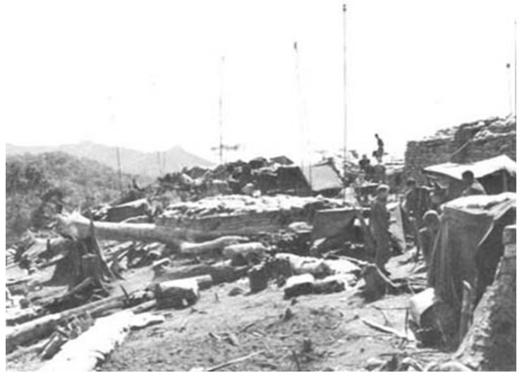
FIRE SUPPORT BASE ON A RIDGE NEAR DAK To. Tall antennas were used to extend range of mobile voice radios.
